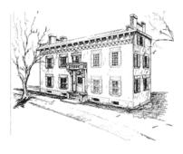
The Jacob Grafius House, 1857, is a Federal-Tuscan Transitional style two-story Flemish bond brick dwelling with a symmetric facade similar in treatment to the L. A. Mackey House. The end gables contain twin chimneys connected with a parapet, and have triple windows at the peak. The most outstanding feature of this building is the highly decorated frieze which has floral designs between closely spaced brackets.
