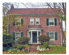
The L. A. Mackey House, 1854, is a Federal-Tuscan Transitional, two-story, Flemish bond brick dwelling with the main section measuring 44.5' by 39.5'. The symmetric facade has five windows across the front, a bracketed cornice with dentils (which is carried along the sides of the building), a decorated frieze with five oblong windows, and a deeply recessed entrance with circular paneled door flanked by side
